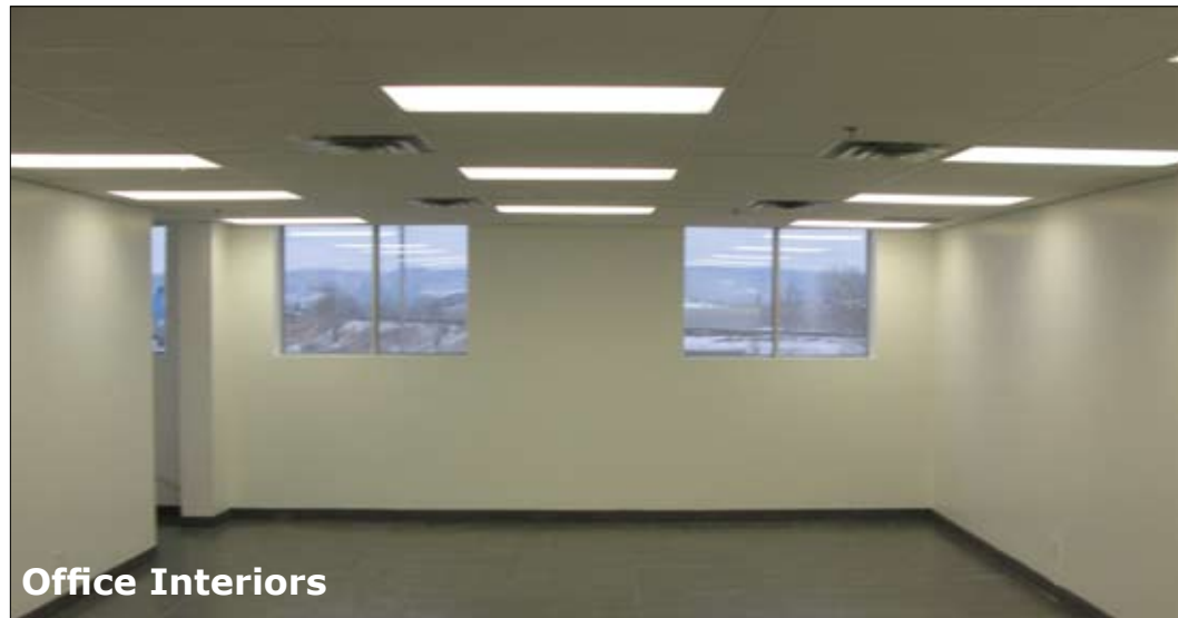
Cervello - Office renovations
